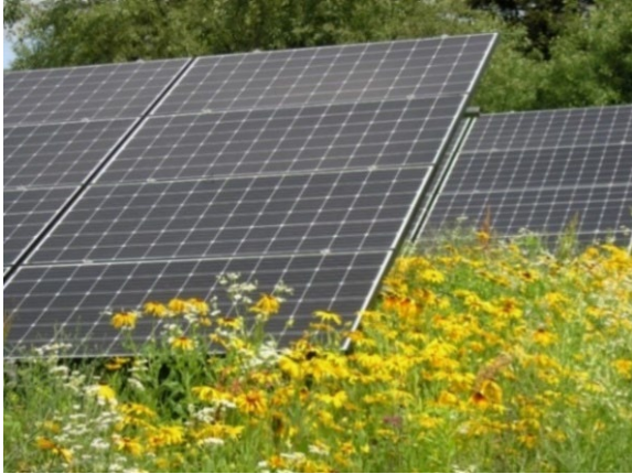
Ground-mounted solar arrays underplanted with pollinator plant species, DEC Stamford Sub-Office (Photo: DEC)
