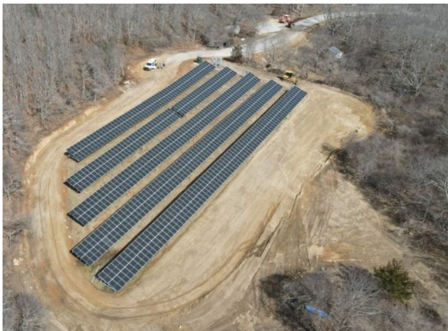
OPRHP staff constructed a 262kW solar array at Hither Hills State Park on the east end of Long Island. The array generates enough electricity to cover the entire park's annual electric usage using renewable energy.
